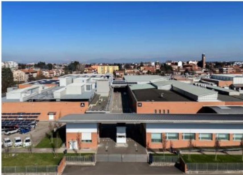
Eurojersey's headquarters and manufacturing facility in Caronno Pertusella, Varese, © Eurojersey
